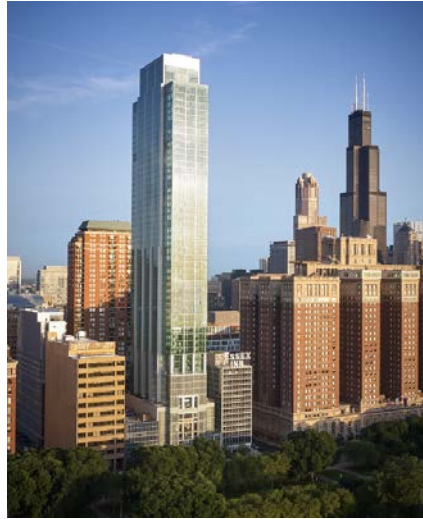
Essex on the Park's Exterior, credit: David Burk (High-resolution photography is available here )
