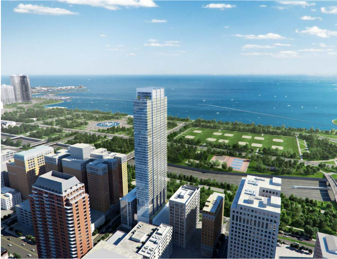
Aerial rendering of Essex of the Park, featuring views of Lake Michigan and Grant Park, courtesy of Oxford Capital Group / Hartshorne Plunkard Architecture
